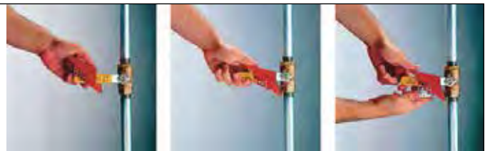
Step 1 Slide on Step 2 Squeeze together Step 3 Apply lock
