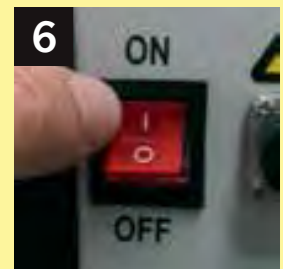
6 Verify equipment isolation
